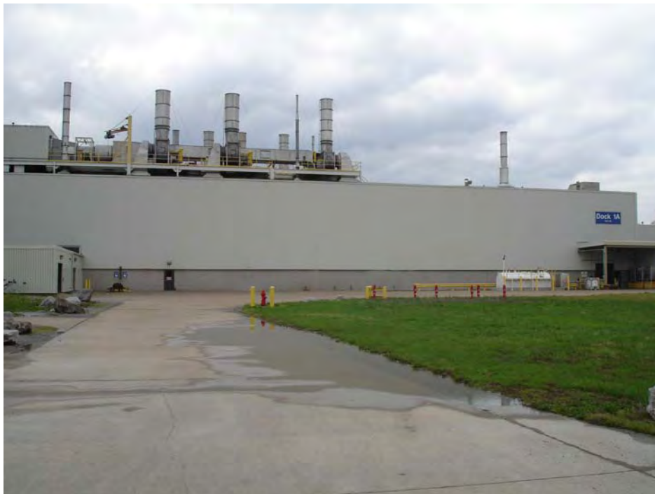
Site for the Potential Fascia Plant Expansion
