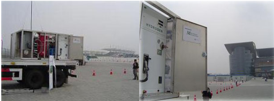
Refuelling system for the Bibendum Challenge in Shanghai (Source: FTI)
