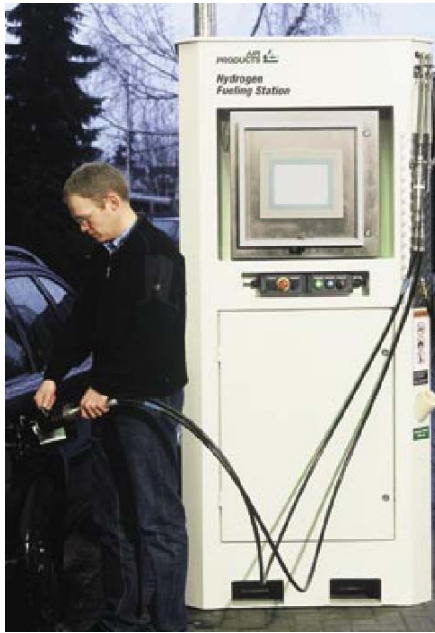
Air Products fuelling station Series 100 (Source: Air Products)
