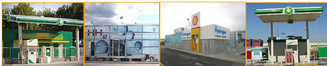
Various fuel cell bus club refuelling stations
