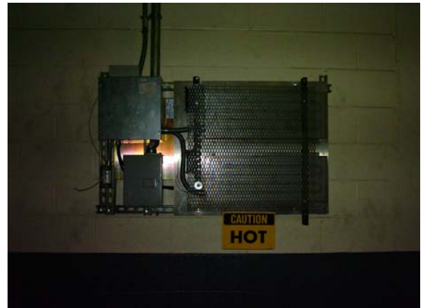
Figure 8 – Test Panel as Installed
