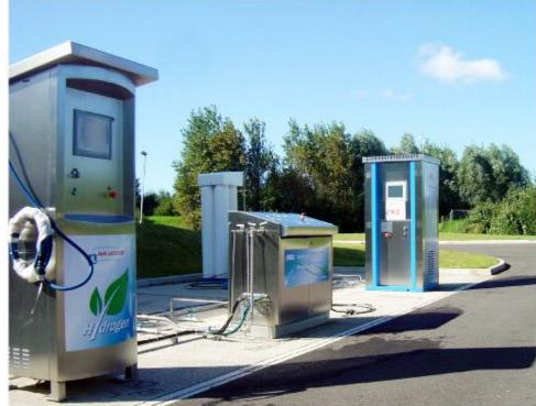
H<sub>2</sub>/CNG fuel dispenser is also installed will allowing mixtures of up to 40% hydrogen in Natural Gas
