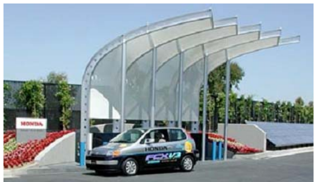
Honda solar powered hydrogen fueling station.
